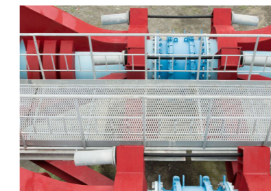
Overhead pipe walkway
